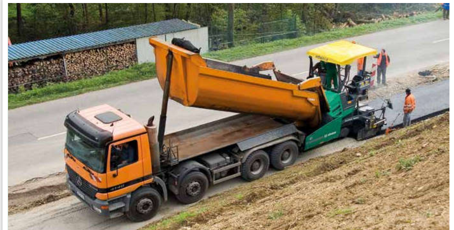
ASPHALT PAVING ON COMBINED FOOT AND CYCLE PATHS
