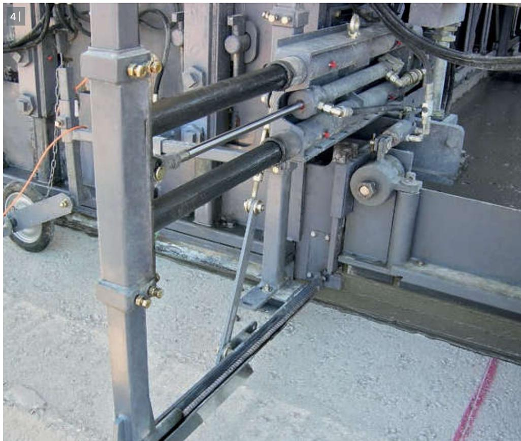
2 | Dowel bars are distributed automatically by means of an intelligently designed chain system.
