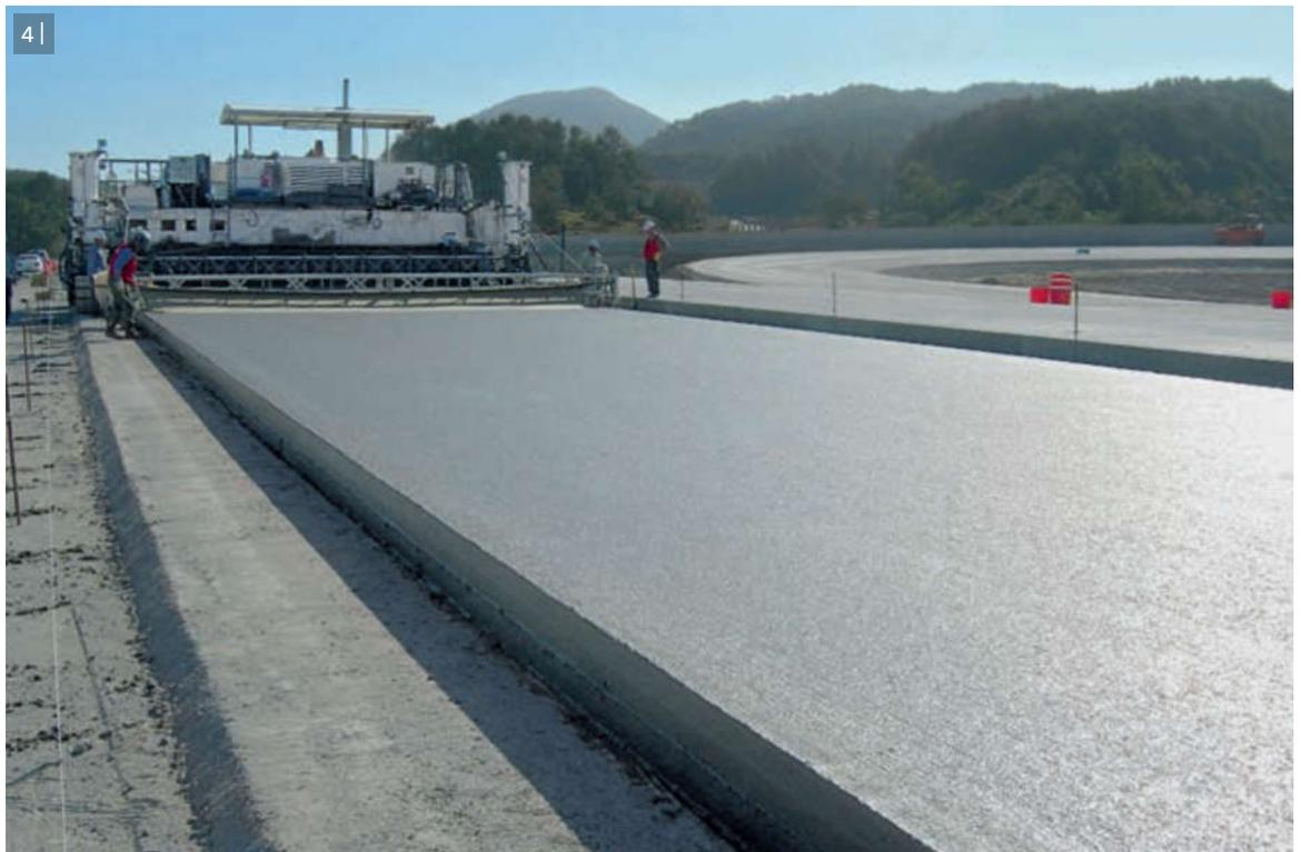
2 | The heavy-duty oscillating beam removes irregularities in the surface across the full width.
