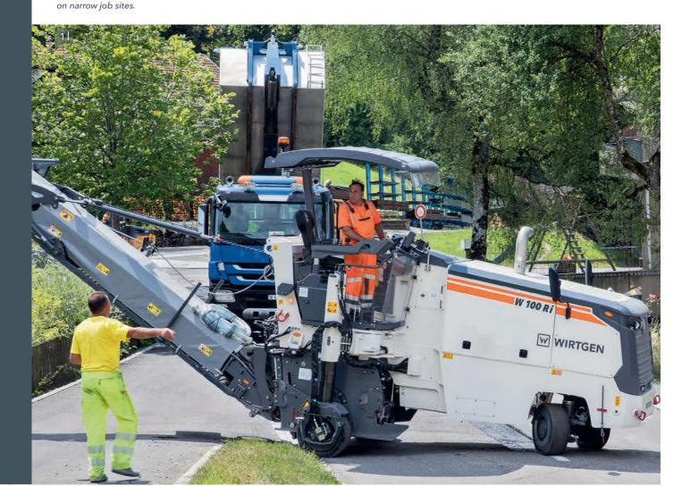
1 The small milling machine excels at fast maneuvering 2 When pivoted in, the right rear wheel makes precise milling along obstacles such as curbs and walls possible.
