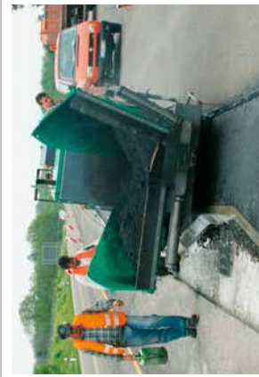
SURFACING MEDIAN STRIPS ON MOTORWAYS
