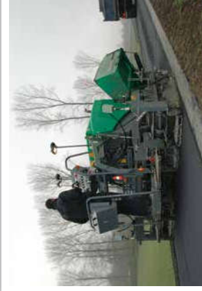
PAVING ASPHALT ON DAMS
