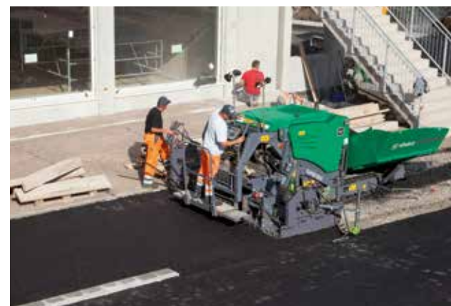
SURFACING LARGE AREAS
