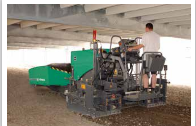
BUILDING THE BASE FOR PAVING SETTS
