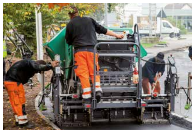
CONSTRUCTING FARM TRACKS
