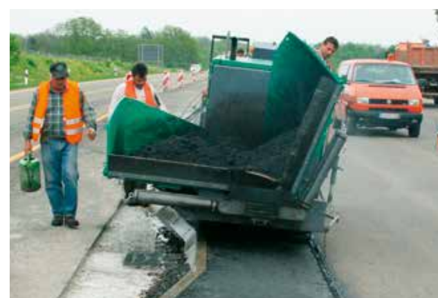
SURFACING MEDIAN STRIPS ON MOTORWAYS
