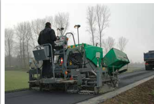
PAVING ASPHALT ON DAMS
