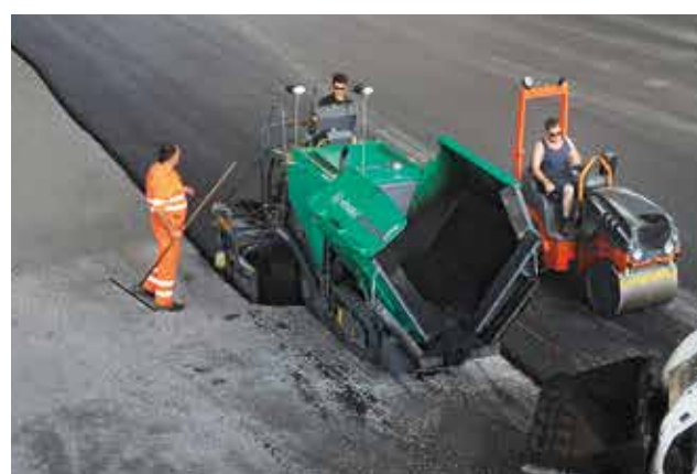
PAVING WORK IN SPORTS FACILITIES
