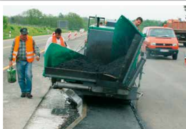
SURFACING MEDIAN STRIPS ON MOTORWAYS
