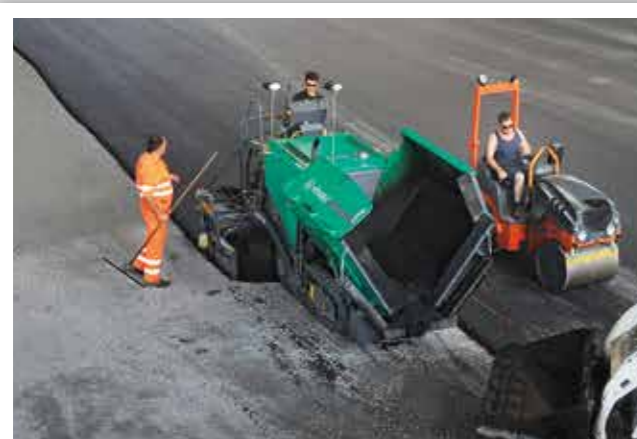
PAVING WORK IN SPORTS FACILITIES
