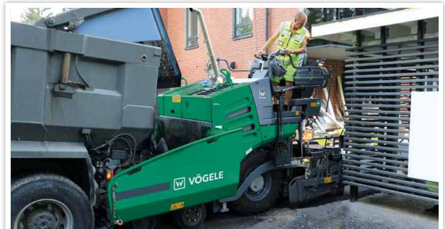
REHABILITATING ACCESS ROADS
