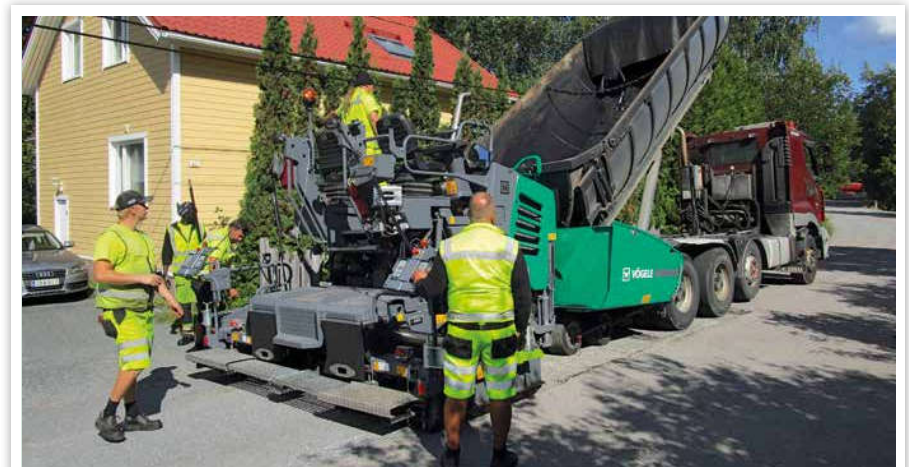
PAVEMENT REHABILITATION ON MUNICIPAL ROADS
