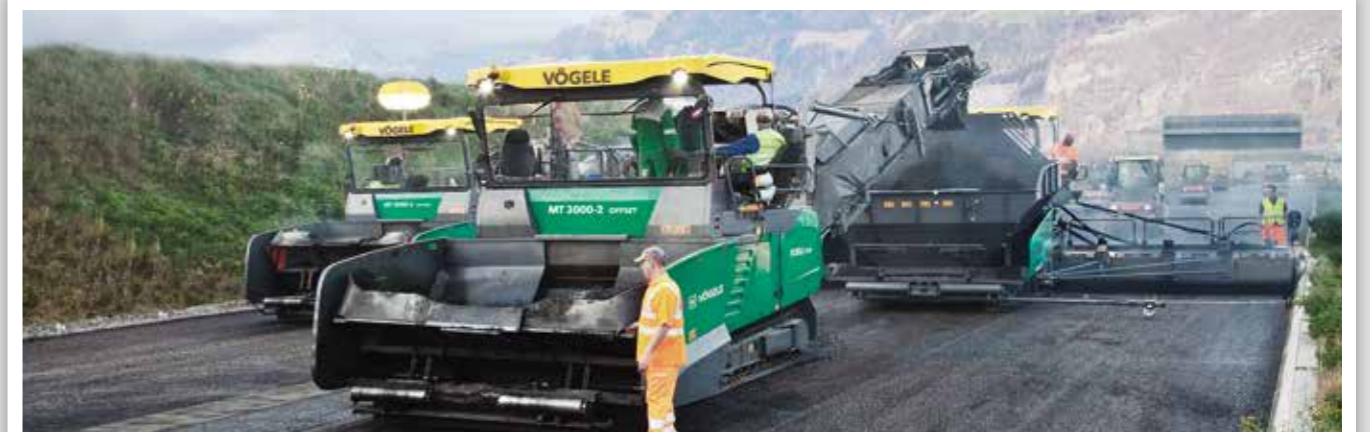
FEEDING PAVERS WHEN WORKING "HOT TO HOT"
