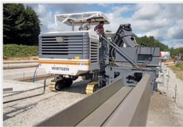
Installation of a special profile for an agricultural operation with the SP 25(i).
