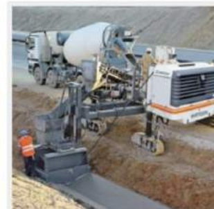
Slipform next to the machine (Offset)
