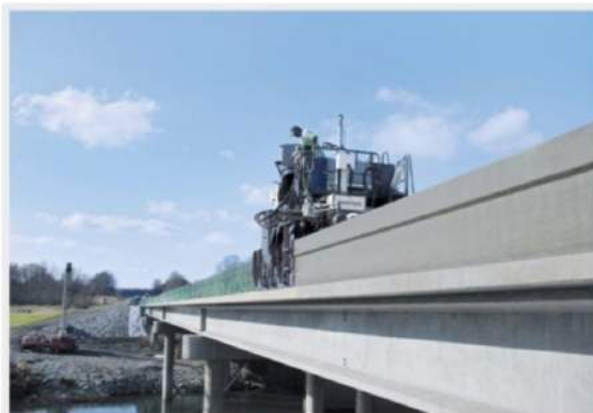
SP 15(i) installs concrete safety barriers on the left-hand side with continuous reinforcement.
