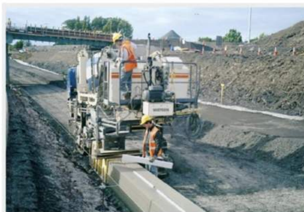
Installation of a slotted gutter for rainwater drainage with the SP 15(i).
