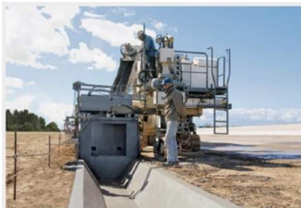
Large water gutters manufactured with the SP 15(i)
