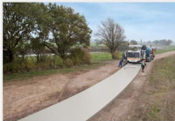
Precise paving of up to 3.5 m wide roads using the WIRTGEN AutoPilot with the SP 25(i).
