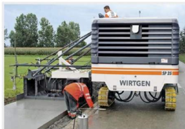
Construction of a 2.5 m wide cycle path with the SP 25(i).
