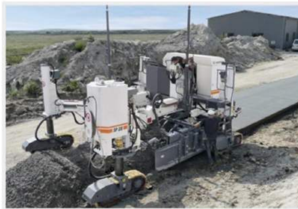
Concrete paving using a 3D control system with the SP 25(i).
